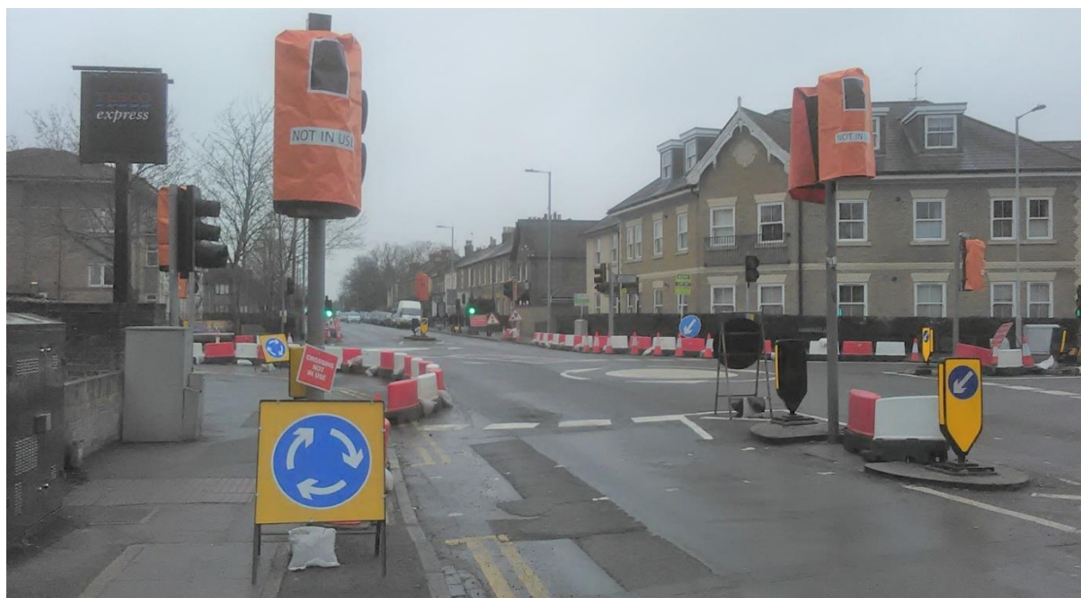
Photo 1: Trial scheme in place. As viewed from Clarence Road looking westwards.
